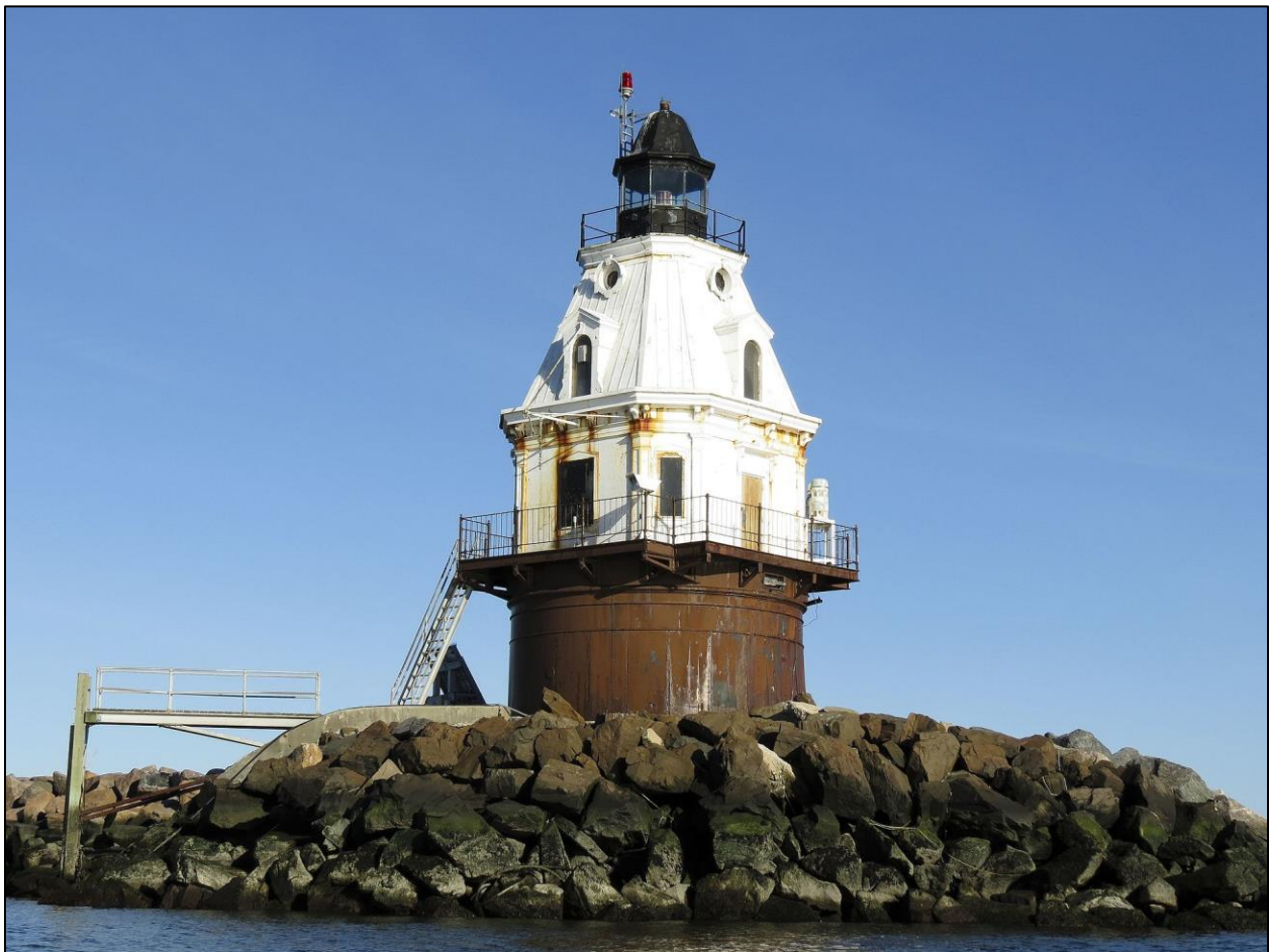
Figure 6: An example of critical infrastructure powered fully by solar energy harvesting. Southwest Ledge Lighthouse in New Haven, CT was fully automated in 1973. The solar panel array is located to the left of the main structure and the energy storage batteries are located on the main level inside the structure. Note the many various loads powered by this system: a primary VRB-25 rotating beacon, an emergency 300mm lantern, both primary and emergency FA-232 fog signals and a VM-100 fog detector – all visible within this image [7].
